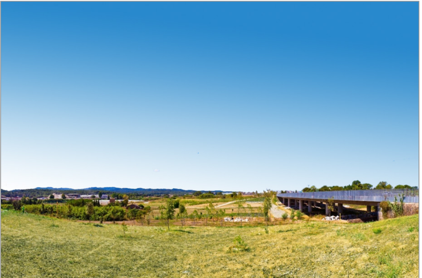
CERDANYOLA-SANT CUGAT BP-1413 ROAD AND ITS WILDLIFE CROSSINGS (TO THE RIGHT)
